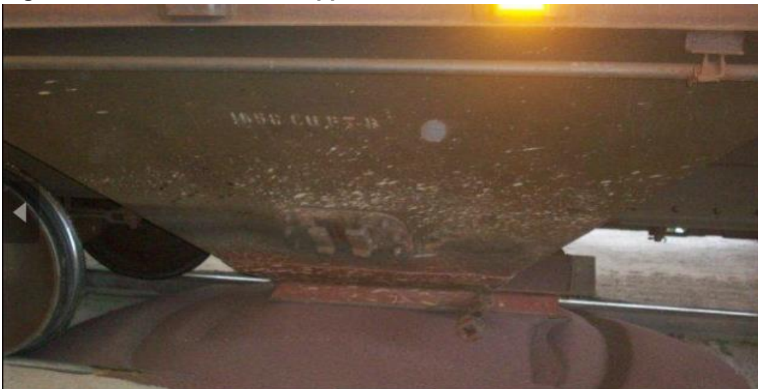
Figure 9 Bottom hatch of a hopper car
